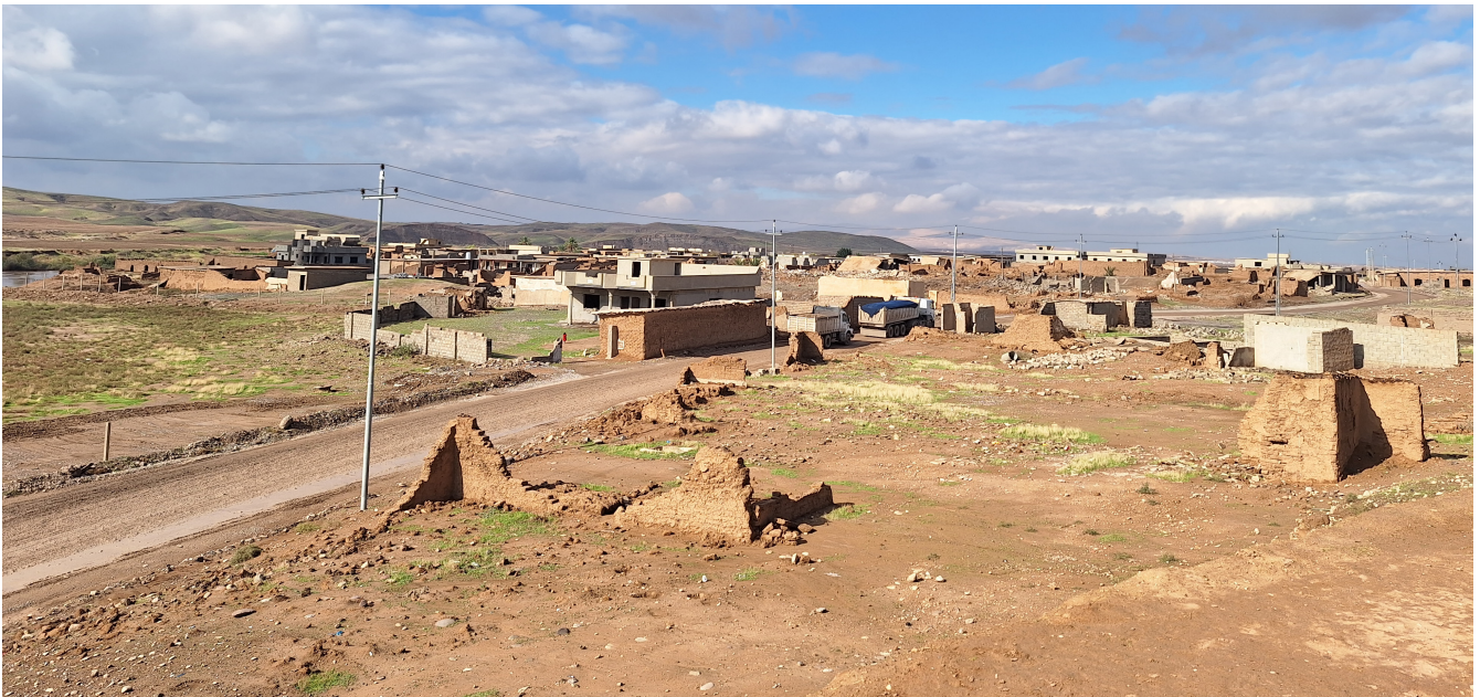
Figure 9: Chamakor Village Electricity Poles on Main Road Not Connected to Village
