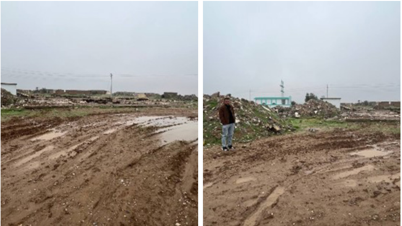
Figure 16: Unpaved External Road in Tal Aswad Kabir
