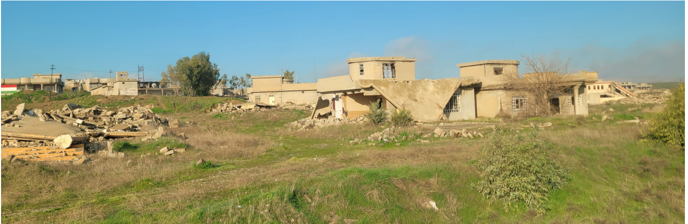
Figure 21: Hasansham Village House Destruction and Debris
