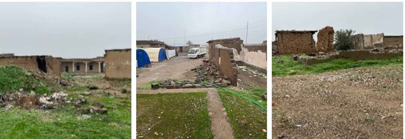
Figure 14: Destroyed Housing and Current Shelter in Tal Aswad Kabir
