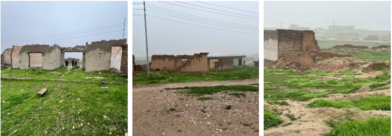
Figure 4: Mangoba Destroyed Housing
