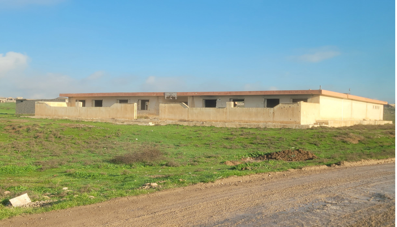
Figure 20: Hasansham Village Primary School with Minor Damage
