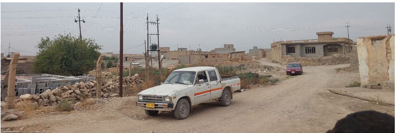
Figure 6: Shirkan Village Electricity Network Cable, Poles, and Internal Road
